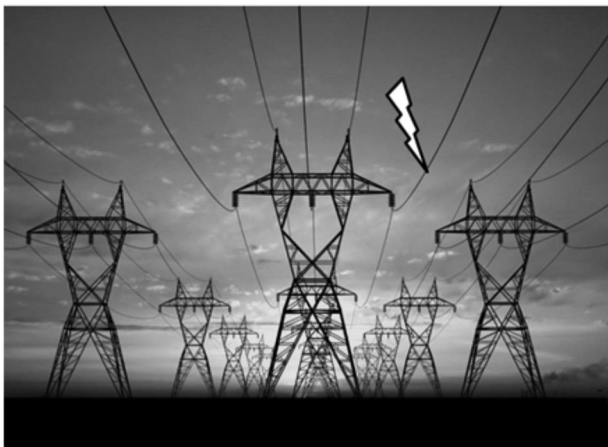
Fig. 3 A Pictorial View of a Typical Long Transmission Line with a Direct Lightning Stroke
