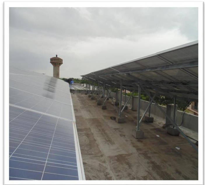
Fig 4(b): Side view of installed solar panels.
